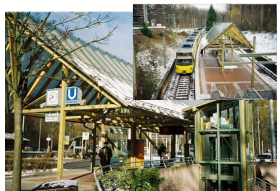
Pictures: Stuttgart Tram Station (Steve Shaw)
